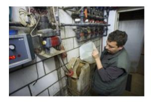
Once the water pipe is uncontaminated, it can be kept clean by adding (a low dose of) disinfect-ants/detergents to the drinking water. [Photo: Van Assendelft]
